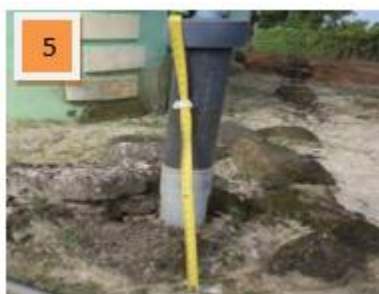
Plate 5: A PVC casing pipe extended above the previous height in a bid to prevent the intrusion of the floodwater contamination. The mark of the white tape indicates the level the floodwaters above the initial casing in that particular location.
