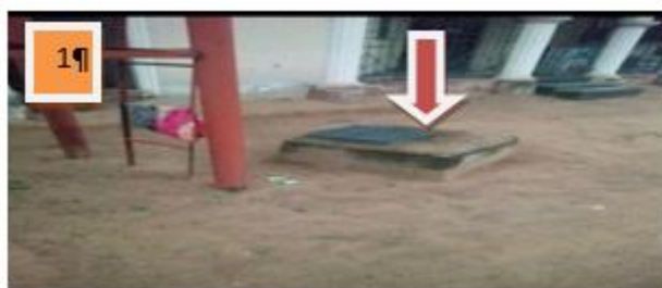
Plates 1 and 2: Borehole casing pipe with submersible pump encased in a concrete slab to prevent intrusion of flood seen in the study vicinity.
