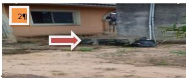
Plates 1 and 2: Borehole casing pipe with submersible pump encased in a concrete slab to prevent intrusion of flood seen in the study vicinity.
